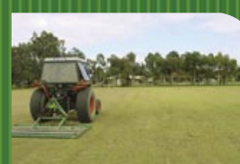
Scott Park Kalamunda final screed to smudge in top dressed soil
